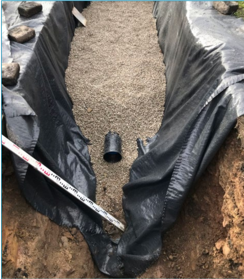
Figure 6: Rain Garden incorporating Liner under Construction
