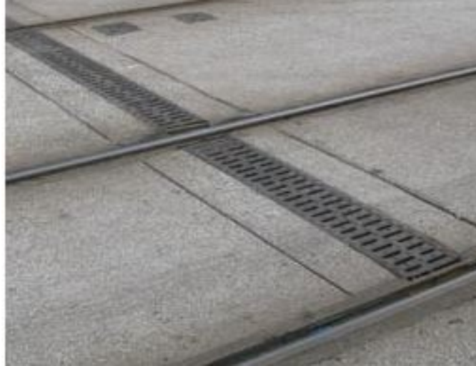
Figure 10: Detail of Slot Drain Collection Channel
